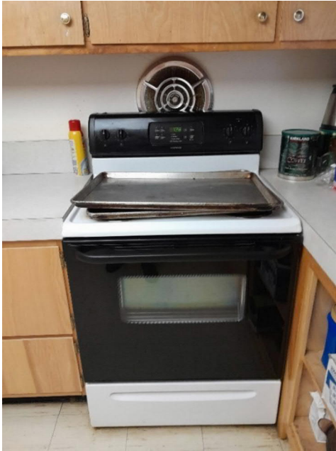
Figure 23 - Kitchen Exhaust Fan
