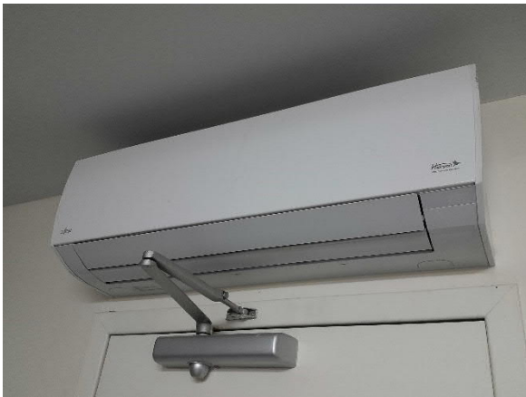
Figure 16 - Heat Pump Indoor Unit
