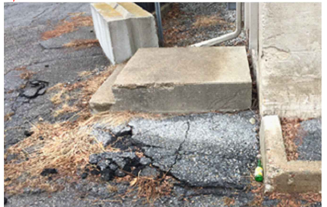
PAVEMENT DAMAGE AND MOVEMENT OF CONCRETE STEPS
