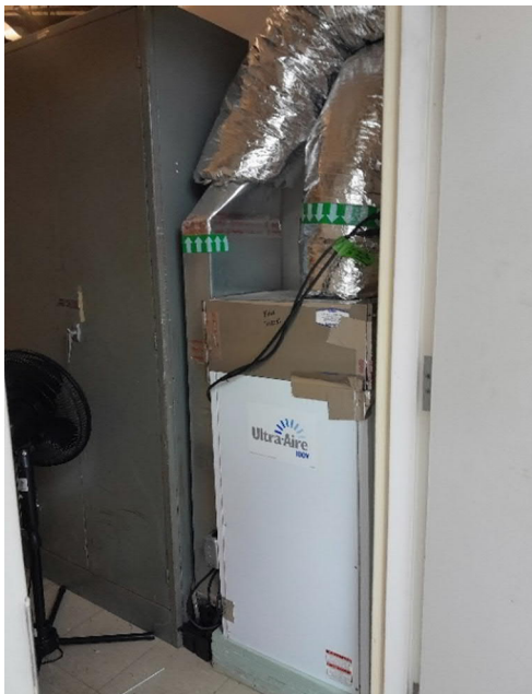
Figure 21 - Ducted Dehumidifier
