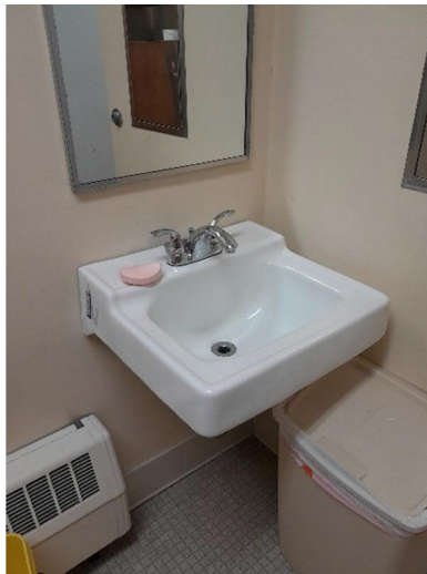
Figure 3 - Mezzanine Restroom Lavatory
