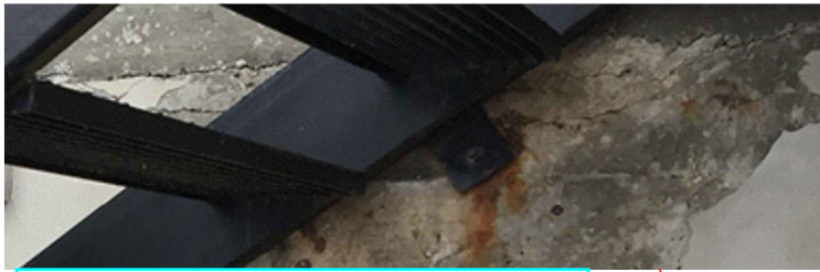
CONCRETE CRACKING AT STAIRS
