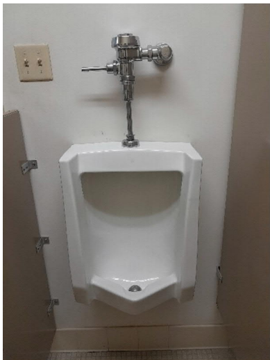
Figure 1 - Mezzanine Restroom Urinal
