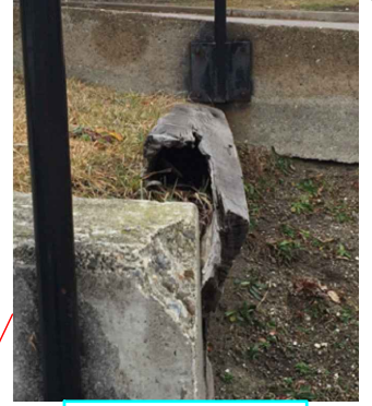
DAMAGED RR TIE SECTION
