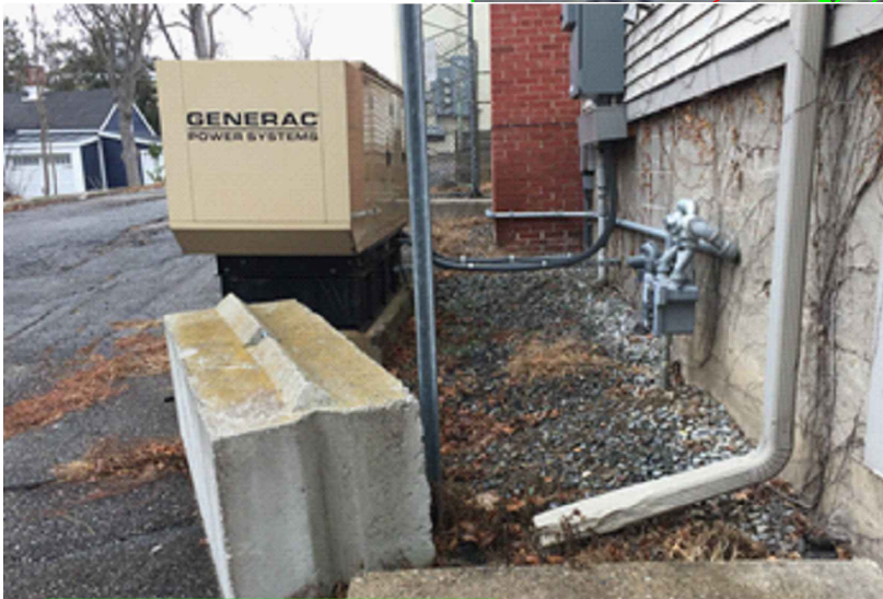
GENERATOR AND OPEN GRADED STONE
